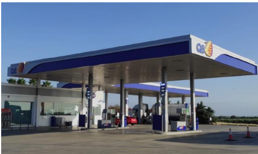
Photo (© Kuwait Petroleum International): The UTA acceptance network now comprises all Q8 stations in Spain
